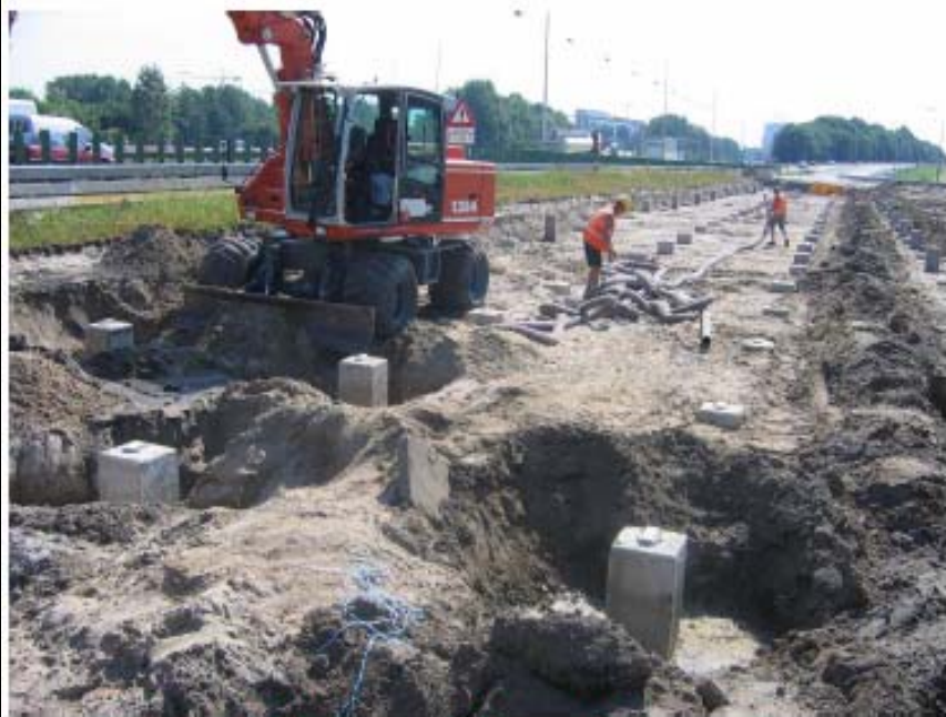
(a) Installation of foundation piles
