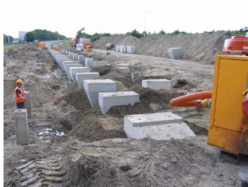
(b) Installation of pile caps on top of piles
